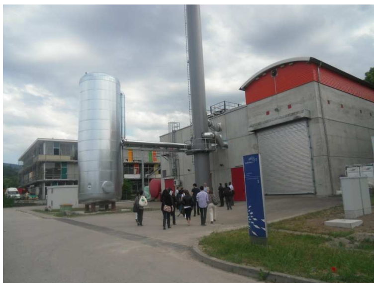
DHC with water storage tank at Vauban
